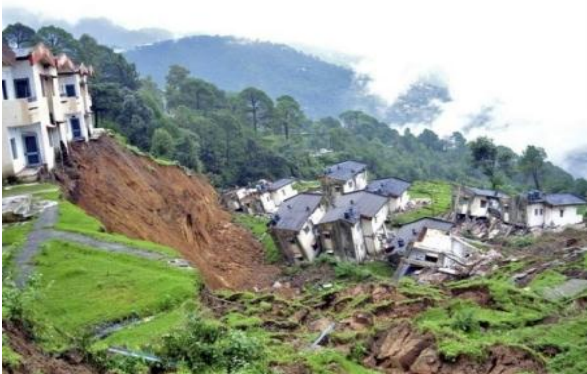
Fig.7. Buildings collapse due to severe landslide at Tirah line
