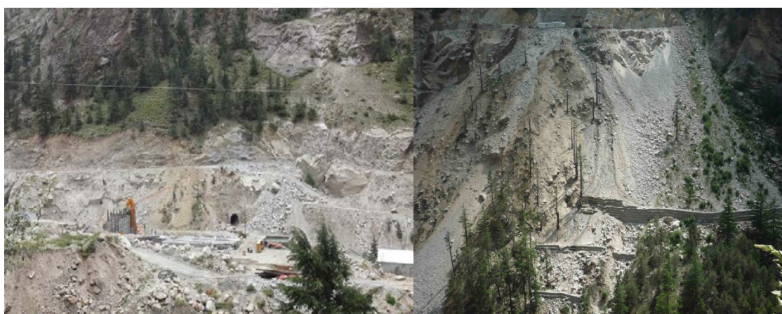
Fig. 7. Land degradation (left) and trees loss (right) during field study near tunnel site of Tidong- I (100 MW) project site
