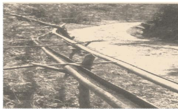
Fig. 5. Bamboo drip irrigation system laid-out in the hilly terrain
