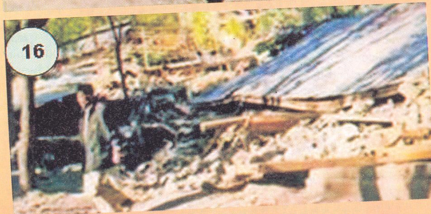
Figs. 14 - 16. Geo-environmental Impact of October 8 Kashmir Earthquake
